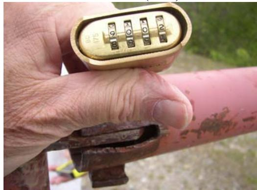
To release/open gate, dial in combination 9002, remove lock and disengage release bar
